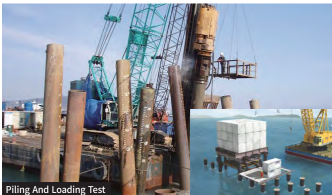
Piling And Loading Test
